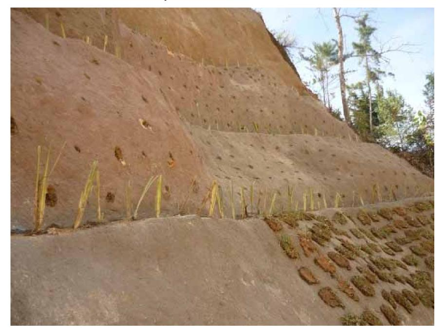
Top rows of vetiver and revegetation being installed on the Mortar
