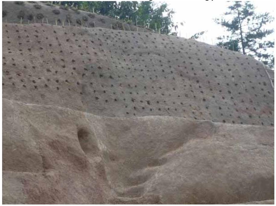
Surface of the EM, It can be seen how the mortar is adapted to the slope topography
